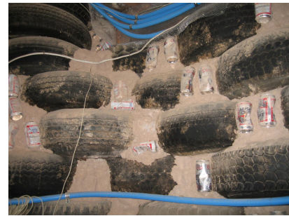
Earthship wall construction
